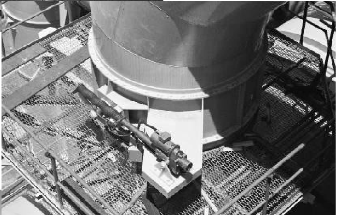
Driving casting-bed dust collection dampers at an iron works. Capacity: 4 ton
